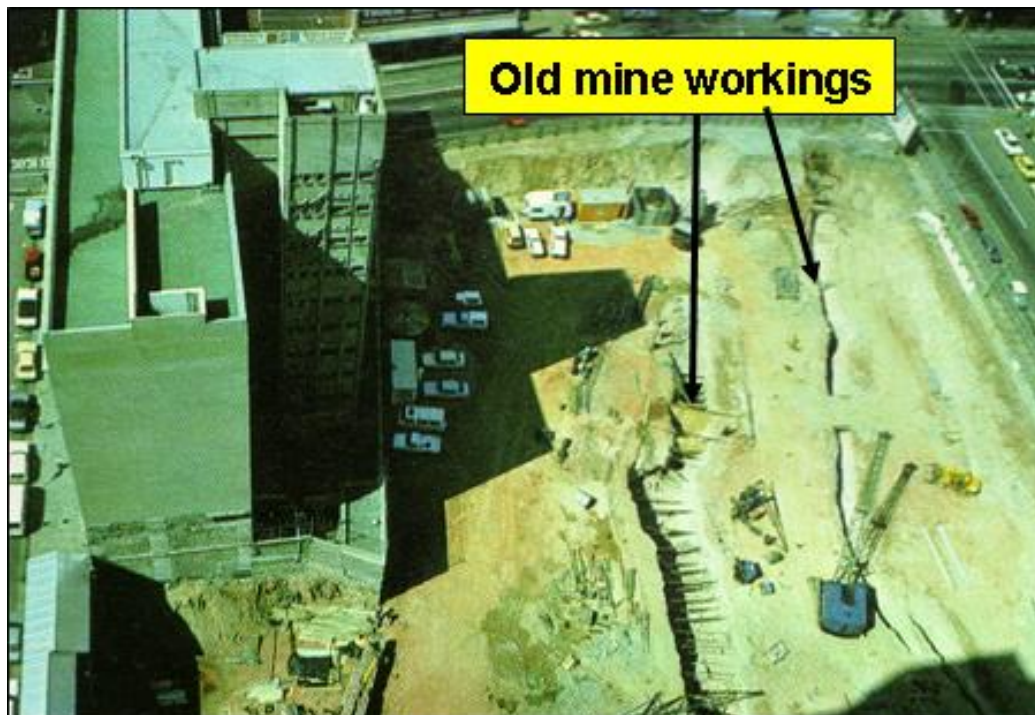
Fig. 8.11: Shallow underground workings of the Ferreira Deep gold mine opened up during excavations for the headquarters of the Priceforbes Federal Volkskas (PFV) at the corner of Sauer and Hall streets in the JHB CBD (early 1980s) (Photo: Editorial Committee, 1986)
